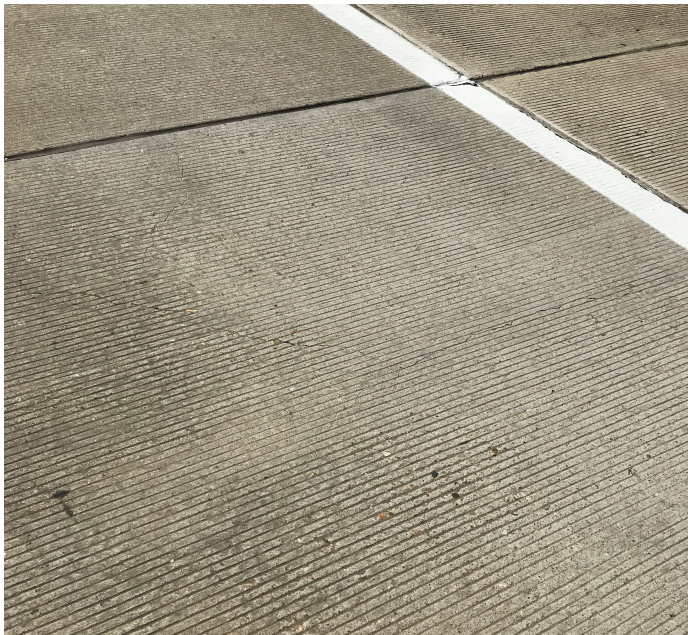
PHOTO 1 Description Deck - Span 1 at Bent 1 left: Diagonal cracking
