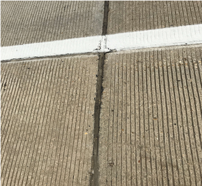
PHOTO 1 Description Joint - Bent 1 : Loss of adhesion
