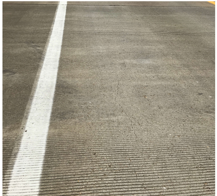
PHOTO 2 Description Deck - Span 1 right : Cracking
