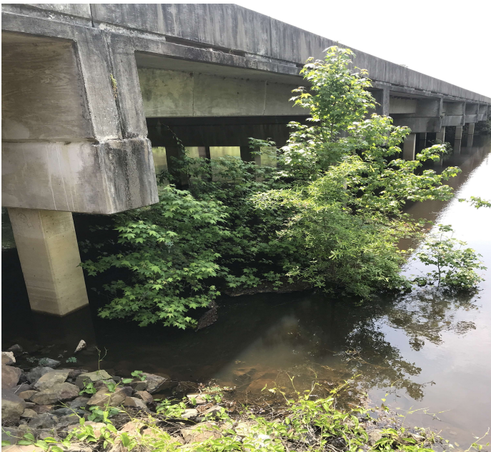
PHOTO 1 Description End-slope - Span 6: Vegetation
