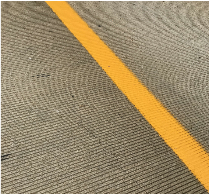
PHOTO 3 Description Deck - Span 4: Cracking
