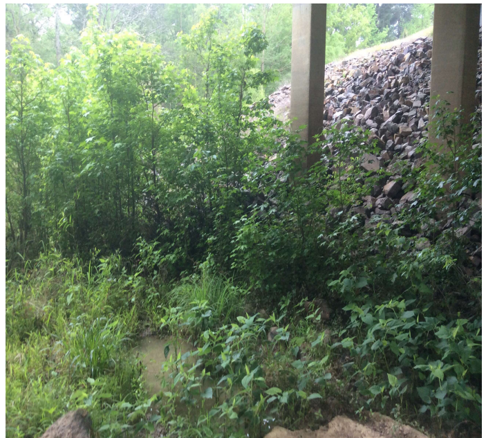
PHOTO 2 Description Span 2 trees and vegetation growing under bridge. Common all spans.
